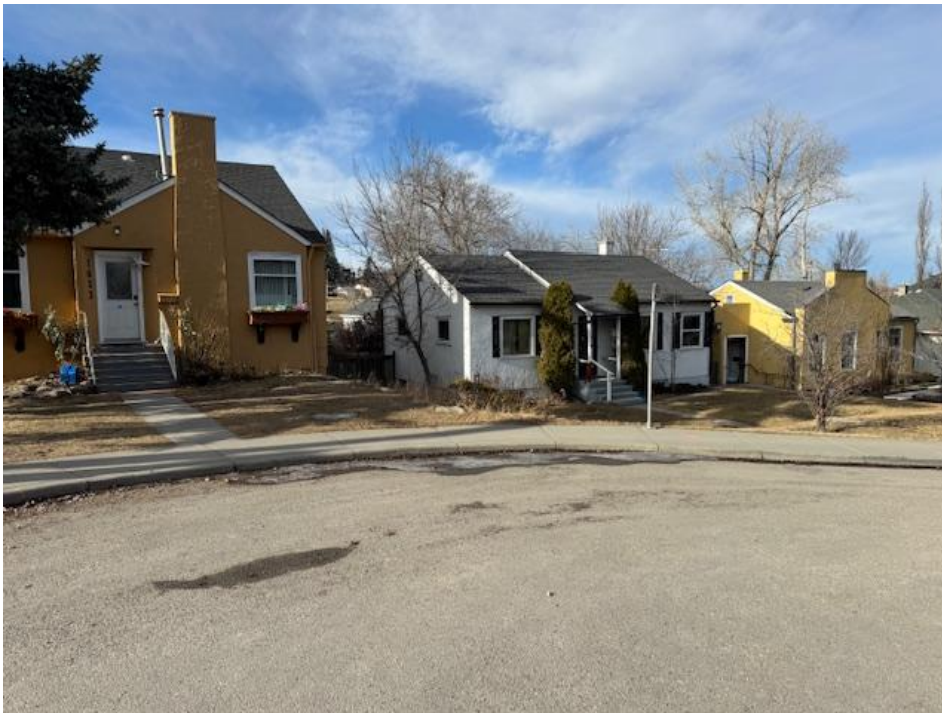
Photo 4: South Elevation of 1619 Summit Street S.W. (subject property) taken from side yard.
