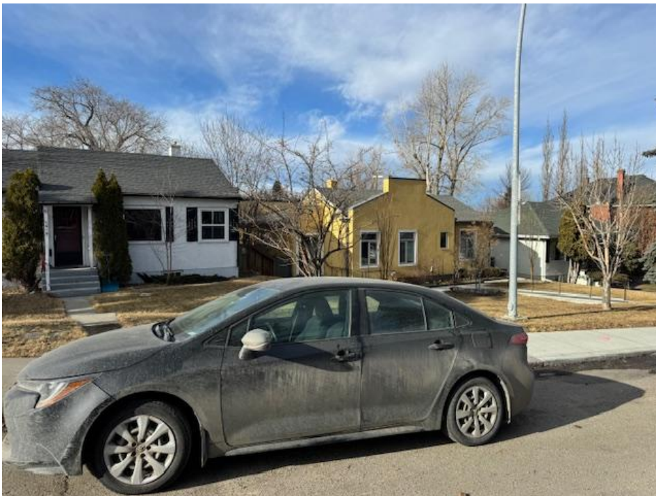
Photo 6: South Elevation of 1615 Summit Street S.W. (North of subject property).
