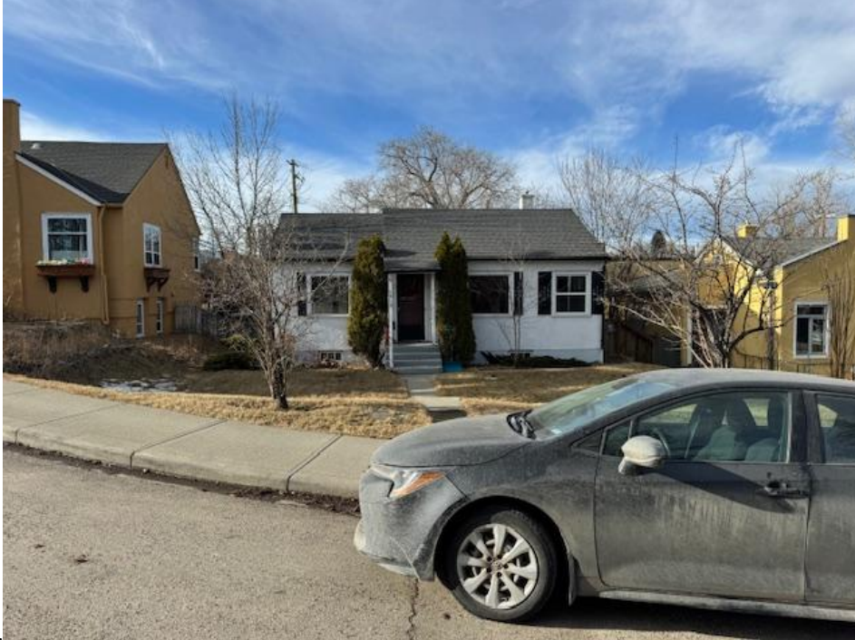
Photo 1: East Elevation of 1619 Summit Street S.W. (subject property) taken from Summit Street S.W.
