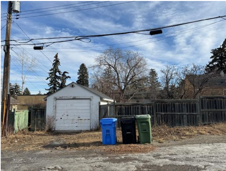
Photo 2: West Elevation of 1619 Summit Street S.W. (subject property) taken from rear lane.
