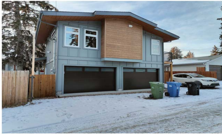
5 REAR VIEW - NORTH NEIGHBOUR - 28 GISSING DR. SW
