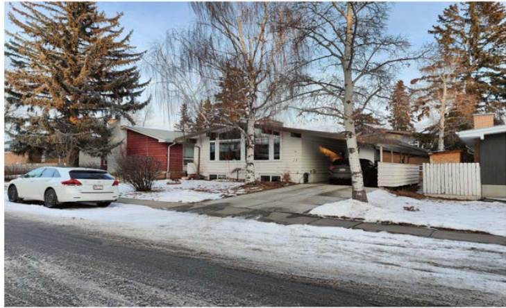
1 FRONT VIEW - NORTH NEIGHBOUR - 28 GISSING DR. SW
