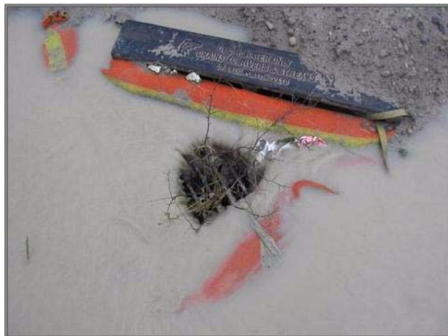
Figure 9-5: Failed Storm Inlet Protection
