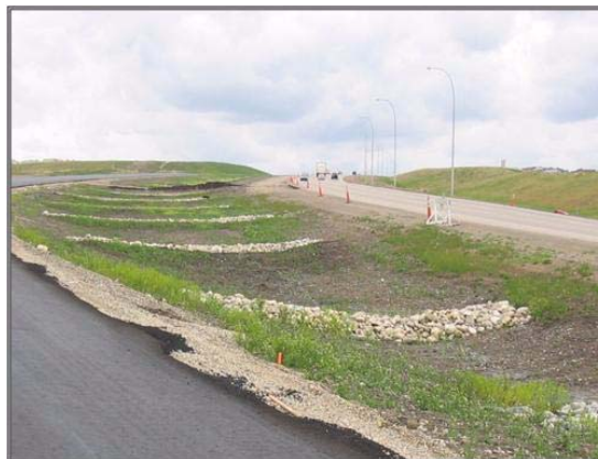
Figure 9-13: Rock Check Dam
