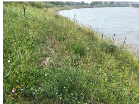
Photo 3-23: High mortality of live cuttings but good herbaceous establishment in void-filled existing riprap installed on the Bow River in 2018 and assessed in 2019 and 2021
