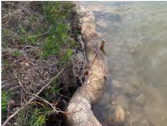
Photo 3-24: Floating wattles at site on the Bow River
