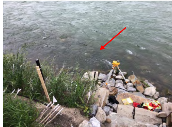
Photo 3-55: Submerged temporary browsing protection fencing in need of repair
