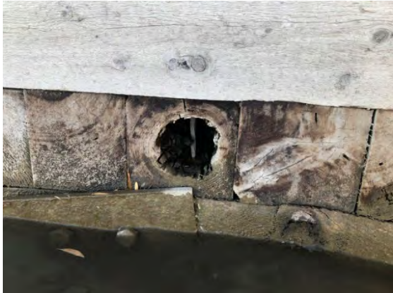
Photo 3-18: Standard grade cedar timber with dry rot used in the timber crib wall
