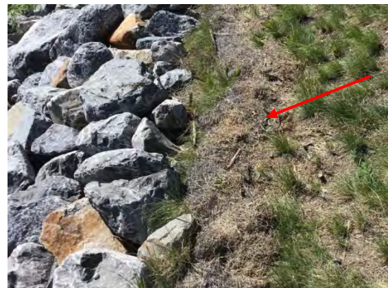
Photo 3-13: Example of biodegradable wattle (Curlex® Sediment Log®) at an advanced state of decomposition installed on the Elbow River in 2015 and assessed in 2018
