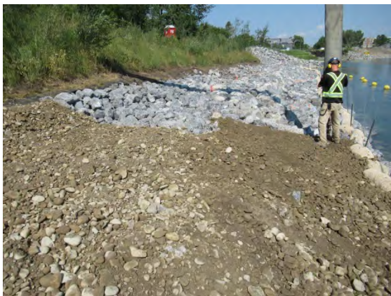
Photo 3-22: Placing planting material in the riprap voids in May 2018
