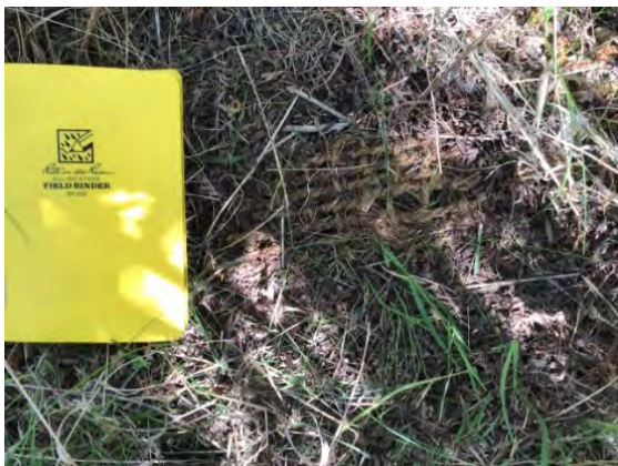
Photo 3-12: Example of biodegradable coir geogrid at a vegetated soil wrap site installed on the Bow River in 2018 and assessed in 2022
