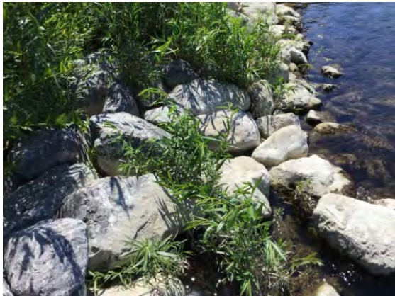
Photo 3-48: Example of root suckering into toe riprap on a site on the Bow River
