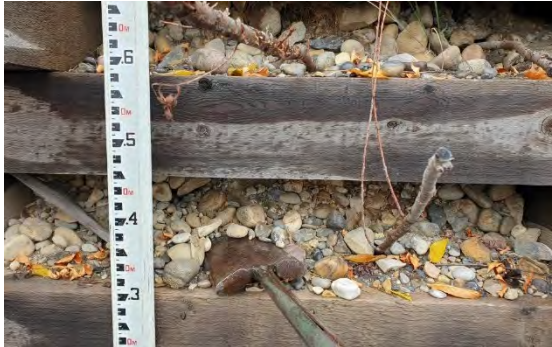
Photo 3-42: Example of dead live cuttings installed on the Bow River in 2016 and assessed in 2019
