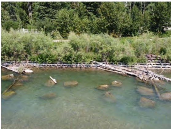
Photo 3-16: Example of fish habitat enhancement boulders and woody debris at a timber crib wall site on the Elbow River assessed in 2019 and 2021
