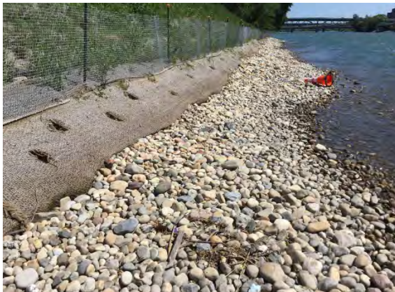
Photo 3-20: Example of riprap covered with river gravels on the Bow River
