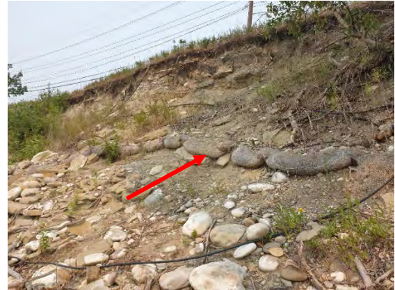
Photo 3-25: Wattle installed improperly and in poor condition on slope with surface erosion
