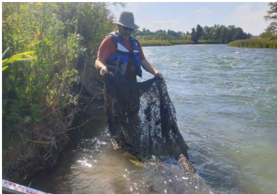
Photo 3-14: Example of synthetic erosion control matting that was installed in 2008 and observed in the Bow River in 2020
