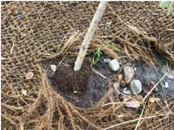
Photo 3-30: Example of TRS installed too shallow on West Nose Creek in 2021 and assessed in 2022
