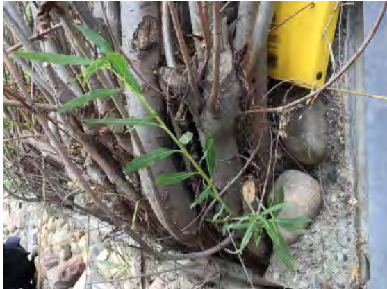
Photo 3-46: Example of stem growth through a structure on the Elbow River
