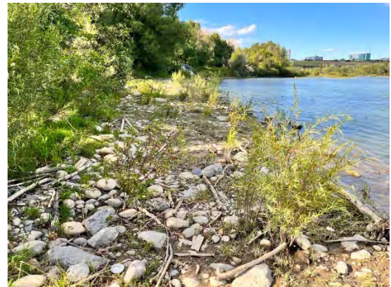
Photo 3-21: Example of void-filled riprap using river gravels and vegetated with live staking on the Bow River
