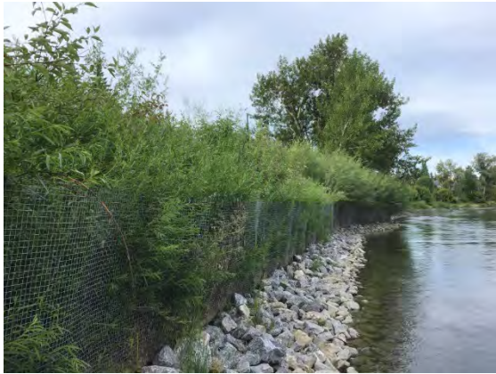
Photo 3-60: Example of a temporary rodent fence installed around a bioengineering site on the Elbow River
