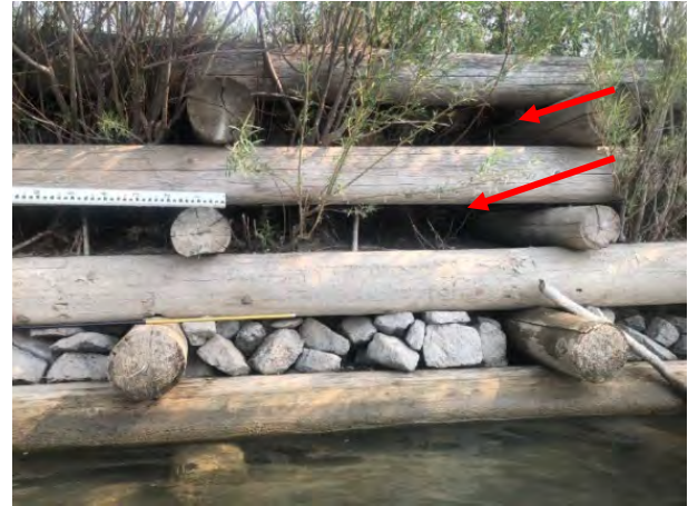
Photo 3-9: Example of backfill material washout in a timber crib wall installed on the Bow River in 2015 and assessed in 2021
