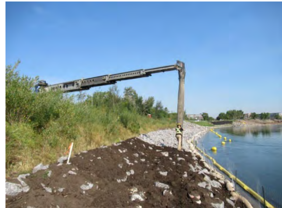
Photo 3-51: Telebelt used to 'shoot' planting material into the void space in existing riprap on a site on the Bow River
