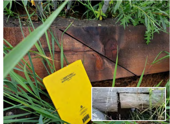
Photo 3-19: Transverse connections between timbers used in the timber crib wall (inset: notched connection for comparison)
