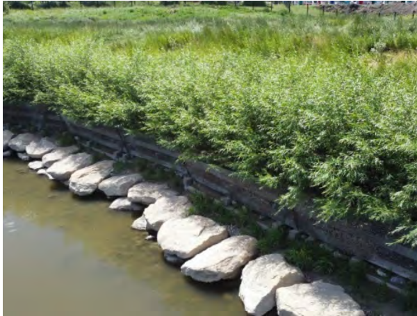
Photo 3-8: Example of stable site with a vegetated timber crib wall installed on Nose Creek in 2021 and assessed in 2022
