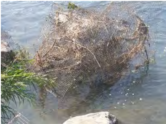
Photo 3-54: Temporary browsing protection fencing to be removed due to hazard to wildlife and the public
