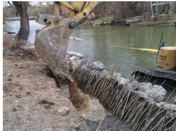
Photo 3-34: Example of long live cuttings placed with 'wet toes' at a vegetated riprap site installed on the Elbow River in 2014 and assessed in 2021
