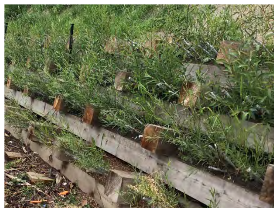
Photo 3-66: Example of a vegetated timber crib wall technique installed on the Bow River in 2019 and assessed in 2020
