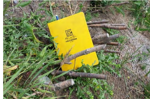
Photo 3-43: Example of dead live cuttings installed on the Bow River in 2018 and assessed in 2019
