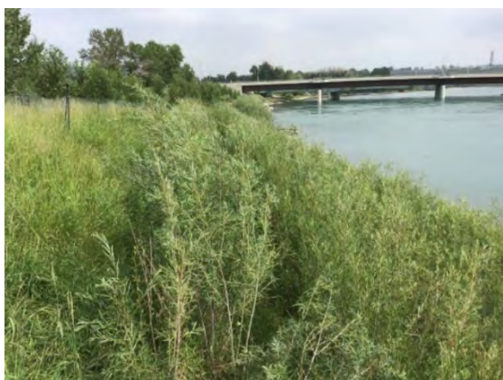
Photo 3-65: Example of a brush layer technique installed on the Bow River in 2018 and assessed in 2019 and 2021
