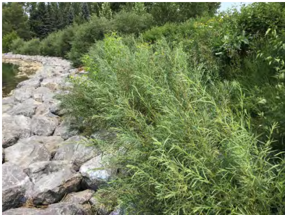
Photo 3-33: Example of good vegetation establishment at a vegetated riprap site installed on the Elbow River in 2015 and assessed in 2021
