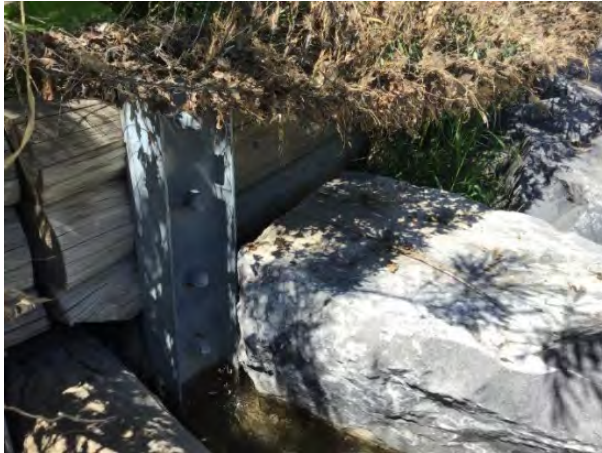
Photo 3-10: Example of site with riprap, timber and steel components installed on the Elbow River in 2015 and assessed in 2022
