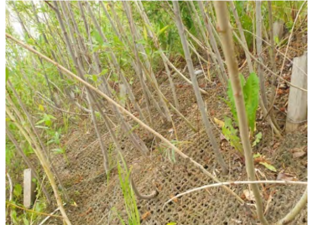
Photo 3-11: Example of biodegradable coir geogrid installed at a site on Bow River in 2017 and assessed in 2019 and 2021
