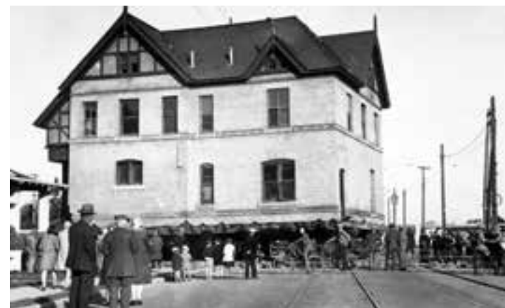
John R. Costigan's house, later occupied by Col. Sam Steele, being moved across 17 Avenue SW from Beltline to its present site in Mission, 1928. W.J. Oliver, photographer. Glenbow Library and Archives Collection, Libraries and Cultural Resources Digital Collections, University of Calgary, CU193180
