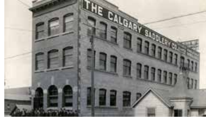
The Calgary Saddlery building, built in 1909 and shown here circa 1915, remains extant at 110–11 Avenue SE. Glenbow Library and Archives Collection, Libraries and Cultural Resources Digital Collections, University of Calgary, CU1207368
