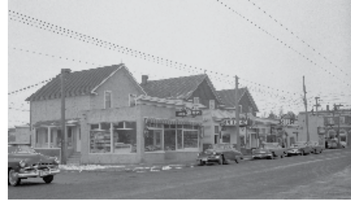
Shops built in front of older homes along 14 Street SW, looking southeast toward 17 Avenue, 1956. Jack De Lorme, photographer. Glenbow Library and Archives Collection, Libraries and Cultural Resources Digital Collections, University of Calgary, CU1140020
