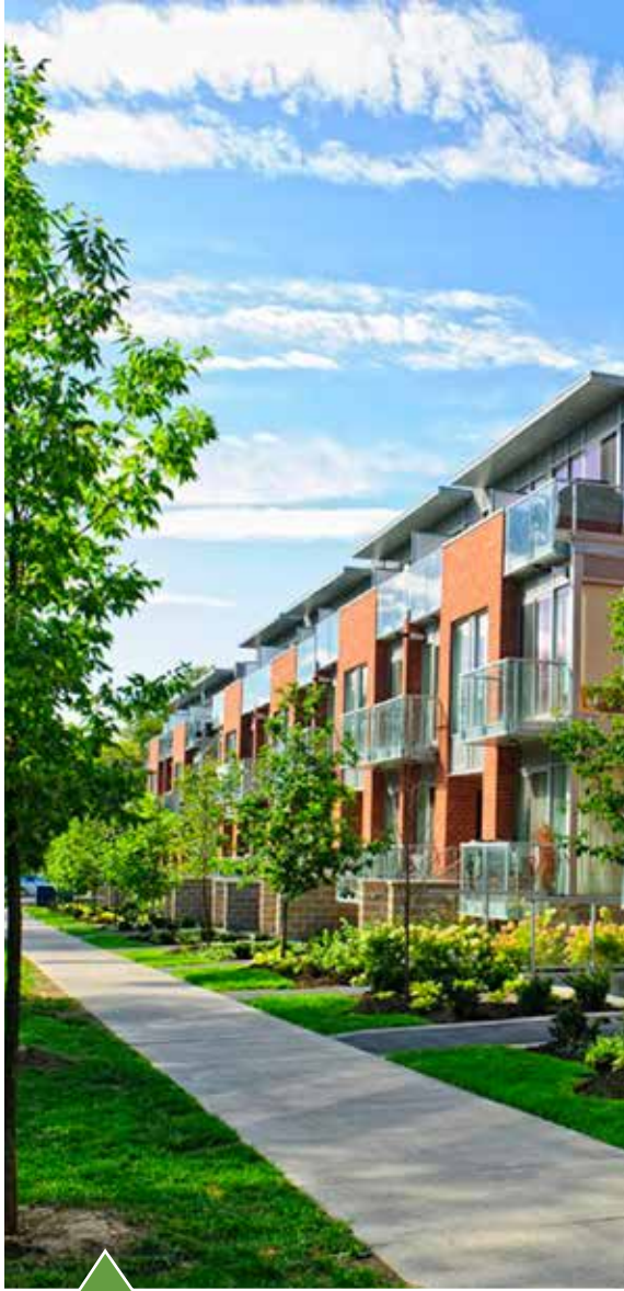
Street-fronting townhomes provide for higher-density development within a form compatible with lower-density adjacent development.
