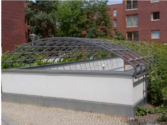
Entrance to a residential underground parkade
