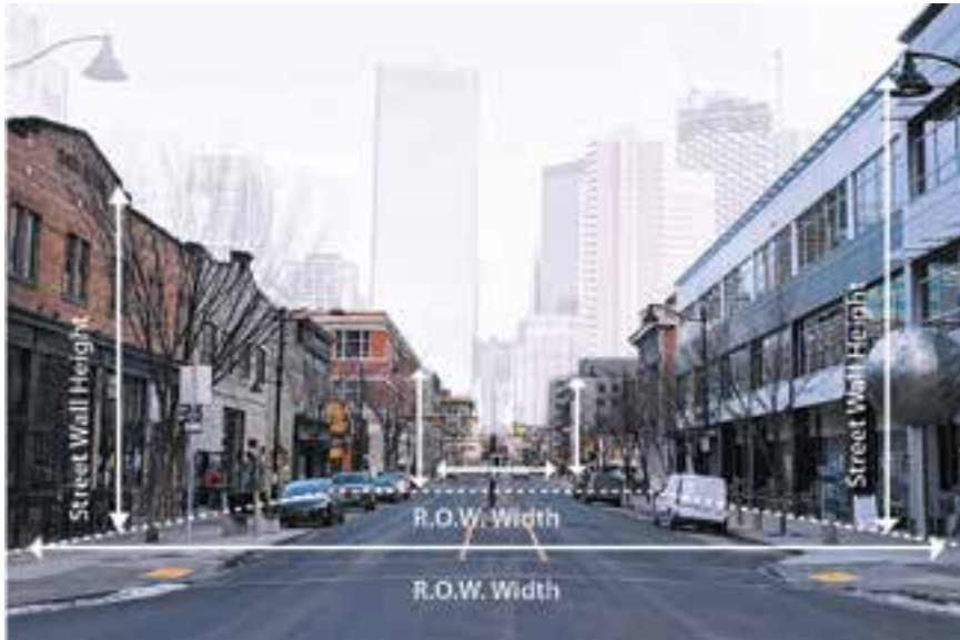
An appropriate street-to-building height ratio is illustrated and supported by policies in the Guidebook.
