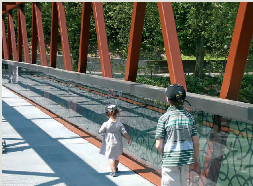
Image 20: Translucent visual marker treatment on a bridge guardrail
